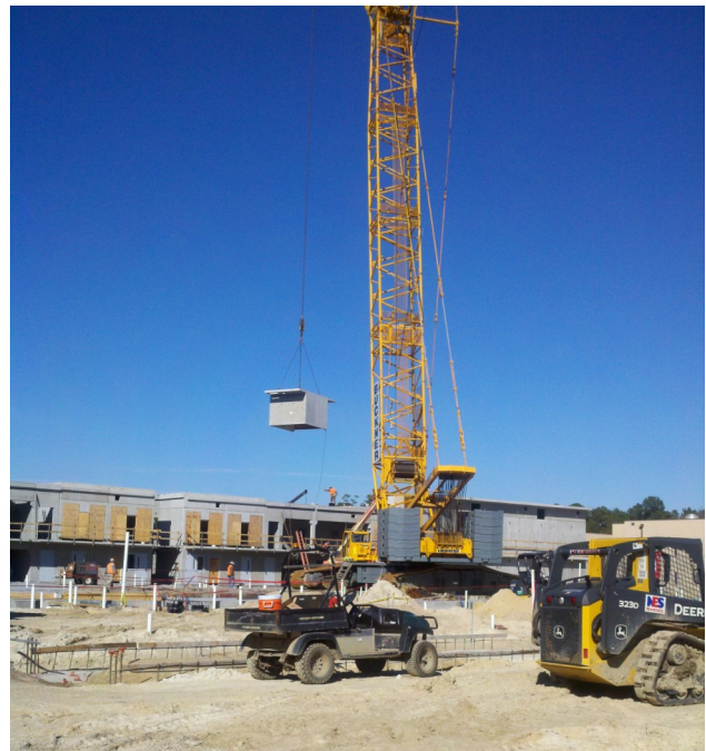
Above: A 600,000 pound crane is stacking more than 500 precast cell modules into place.
